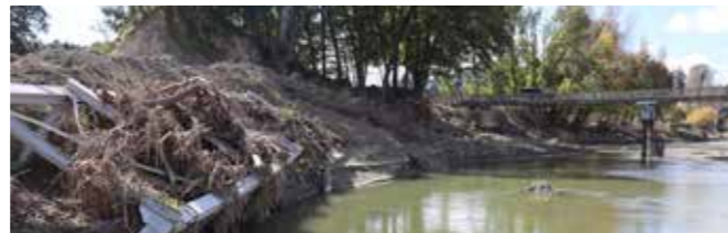
Rissington - old temporary bridge foreground, new temporary bridge background
